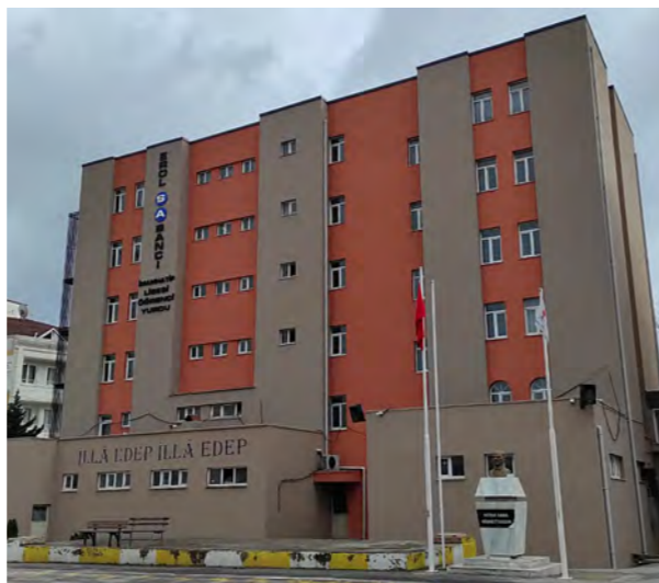
Erol Sabancı Student Dormitory, Kocaeli
